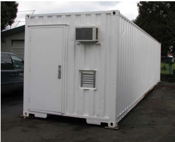
Figure 3. Insect rearing facility modified from a 40 ft marine transport container. Photo Dave Holden
